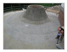
and the third uses soldier bond. The finished roof is extremely strong and can take the loads of the overlying layers of insulation, earth and turf without any stresses to the structure.
