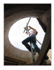
Radiating out from the central pole are springing lines at regular intervals around the circumference. In between each of the formers a cintrel<sup>3</sup> is used.
