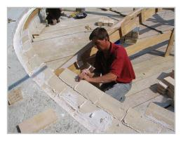
The shape that this first layer has to achieve is shown by 2 types of formwork. The first layer is fixed using plaster to hold the tiles in place.
