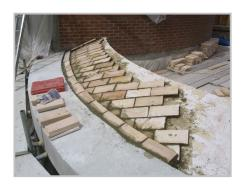
Each layer is built using a different bond. The first layer uses stretcher bond, the second has the tiles laid at a 45° angle
