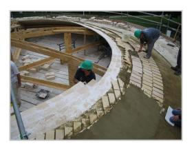
Heavier grog tile is used for the 2<sup>nd</sup> and 3<sup>rd</sup> layers. Both these layers are fixed using cement mortar and are fixed directly on top of the first layer
