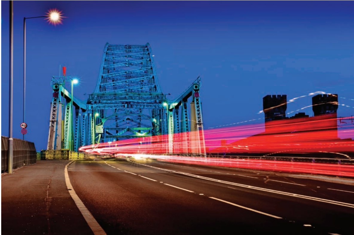
Runcorn Bridge uses an innovative cathodic protection system, with remote monitoring, to stop corrosion and simplify future maintenance and inspection.
