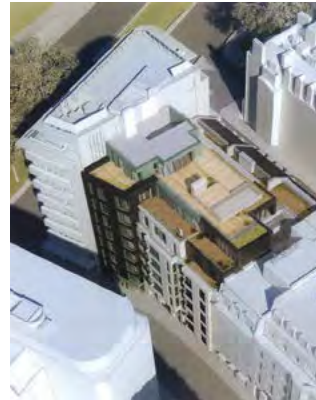
RESIDENTIAL Stanhope Gate – 20 Flats £80,000,000
