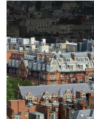
HOTEL, LEISURE & SPORT Claridges Hotel – Redevelopment £19,000,000
