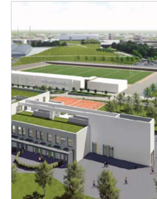
HOTEL, LEISURE & SPORT Park Community Arena – Olympic Legacy Park £10,500,000
