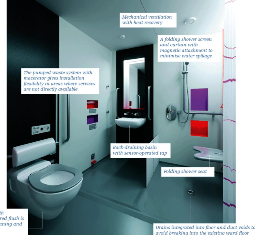
Wall-hung accessible WC with concealed cistern and infrared flush is designed to allow easier cleaning and infection control
