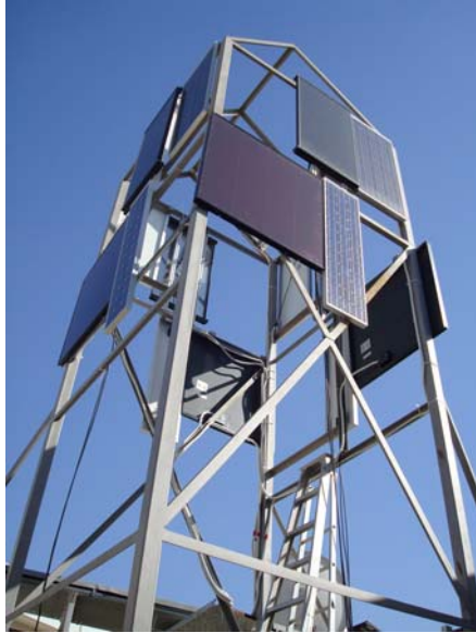
APReS (Atkins Photovoltaic Research Station)
