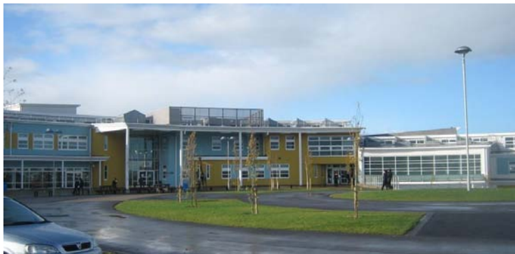
Fig 16: Staff at Kenton School thought the colourful curved façade drew people towards the entrance.
