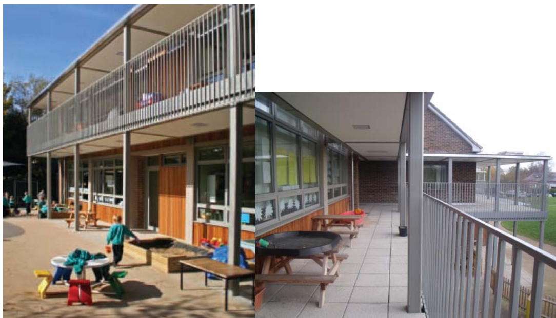
Fig 9: The outdoor learning spaces at Burnham Copse Primary School help to control the classrooms thermal comfort.
